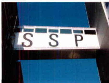
Fig. 1. Gangway SSP connecting the R&D-building E-38 with SSP tower E-52
