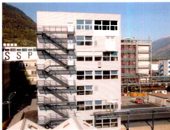
Fig. 2. SSP tower in close proximity to the adjacent launch plant and R&D center
